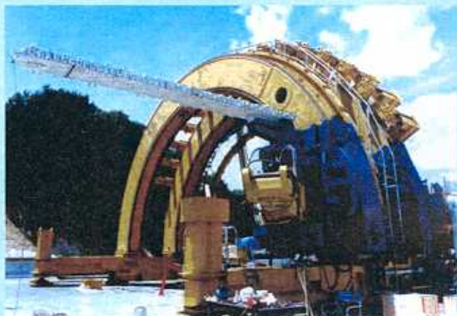
Above: The machine utilises precutting technology using the saw in the photo foreground
