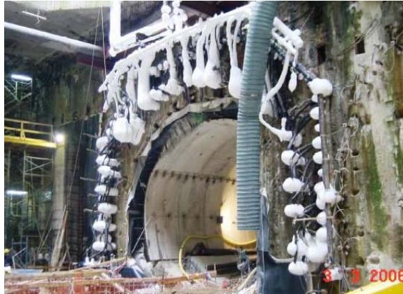
Photo 5. Freezing using nitrogen
