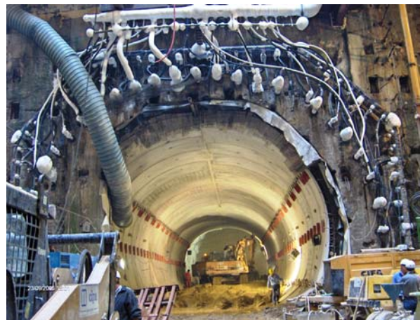
Photo 7. Platform tunnel – Garibaldi Station – Traditional excavation in frozen ground
