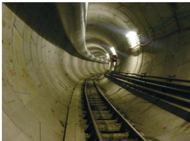
Photo 2. Line tunnel driven using mechanised excavation
