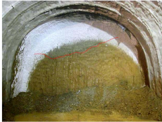
Photo 6. Excavation of the platform tunnels under freezing conditions
