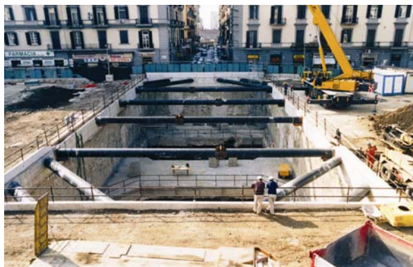
Photo 3. View of the Garibaldi station shaft.
