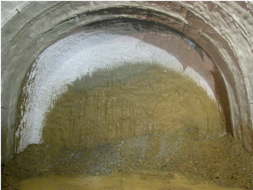
Fig. 13 Face in tuff with freezing of a substantial thickness of ground clearly evident
