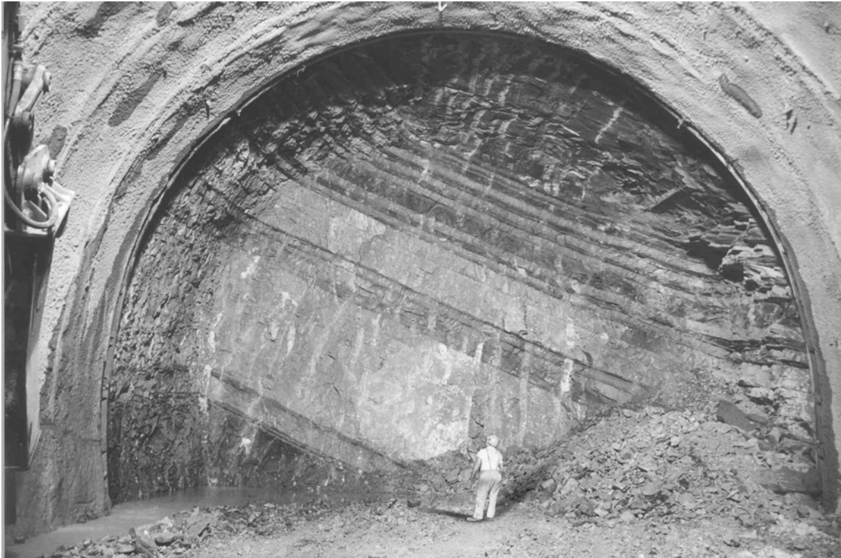
Figure 7. The face of the Vaglia tunnel in the Monte Morello Formation (limestones, marls and sandstones )
