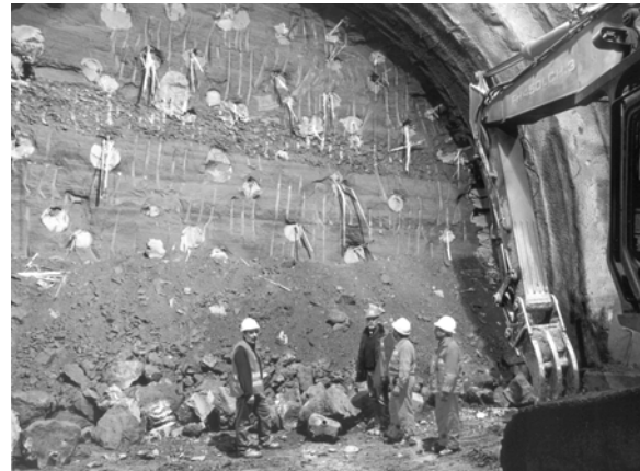
Figure 6. Firenzuola tunnel: the face reinforced with fibre glass structural elements inserted into micro jet-grouted columns
