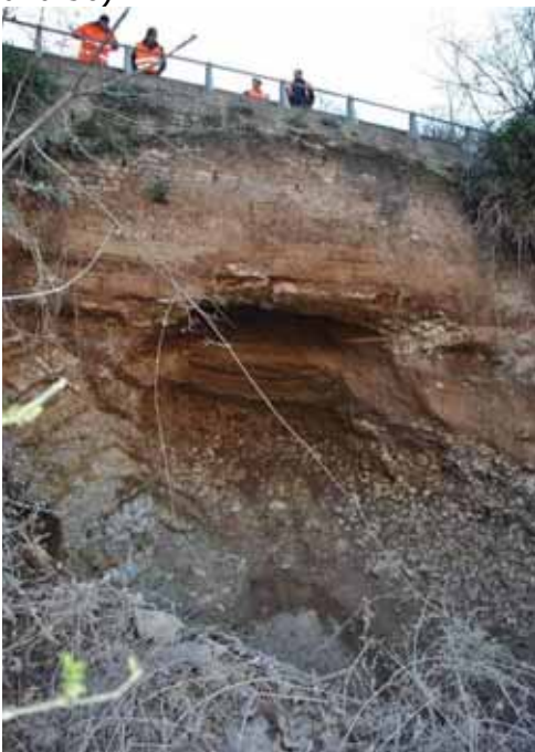
Pic. 5a Overground gap, downstream the SS 77 (detail)
