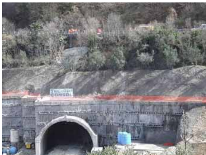
Pic. 5b Overground gap, downstream the SS 77 (general view)
