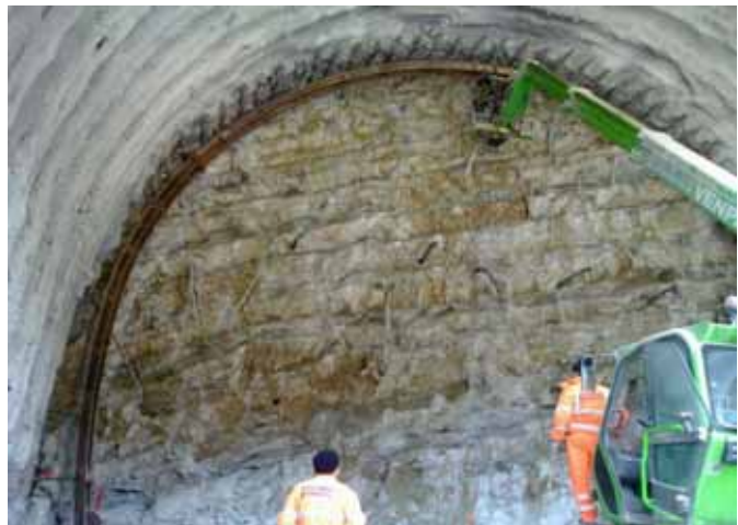
Pic. 3 Rock face at the pk. 4+933 of the Northern bore
