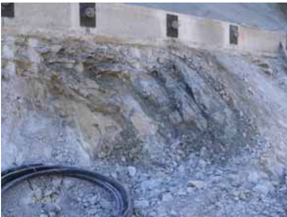
Pic. 2a Maiolica in the bulkhead head beam
