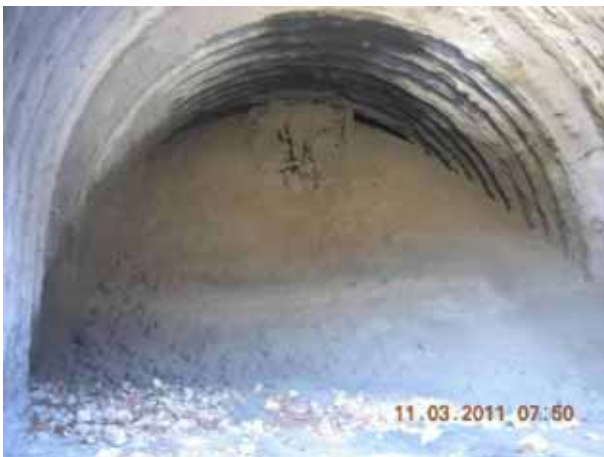
Pic. 4 Material flowed into the tunnel
