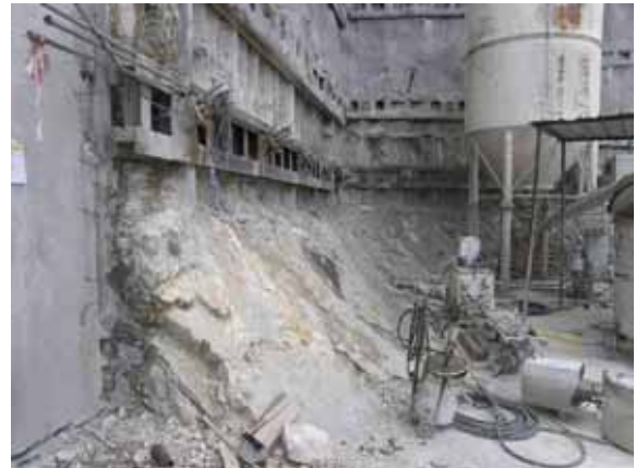
Pic. 2b Maiolica at the base of the bulkhead
