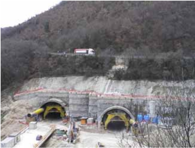
Pic. 1 The "Pale" tunnel. Portal facing Foligno
