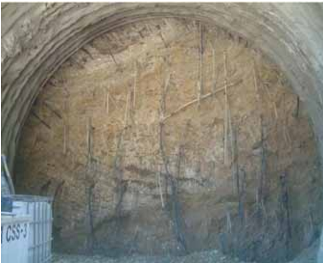
Fig. 6 Debris material at the face of South tube
