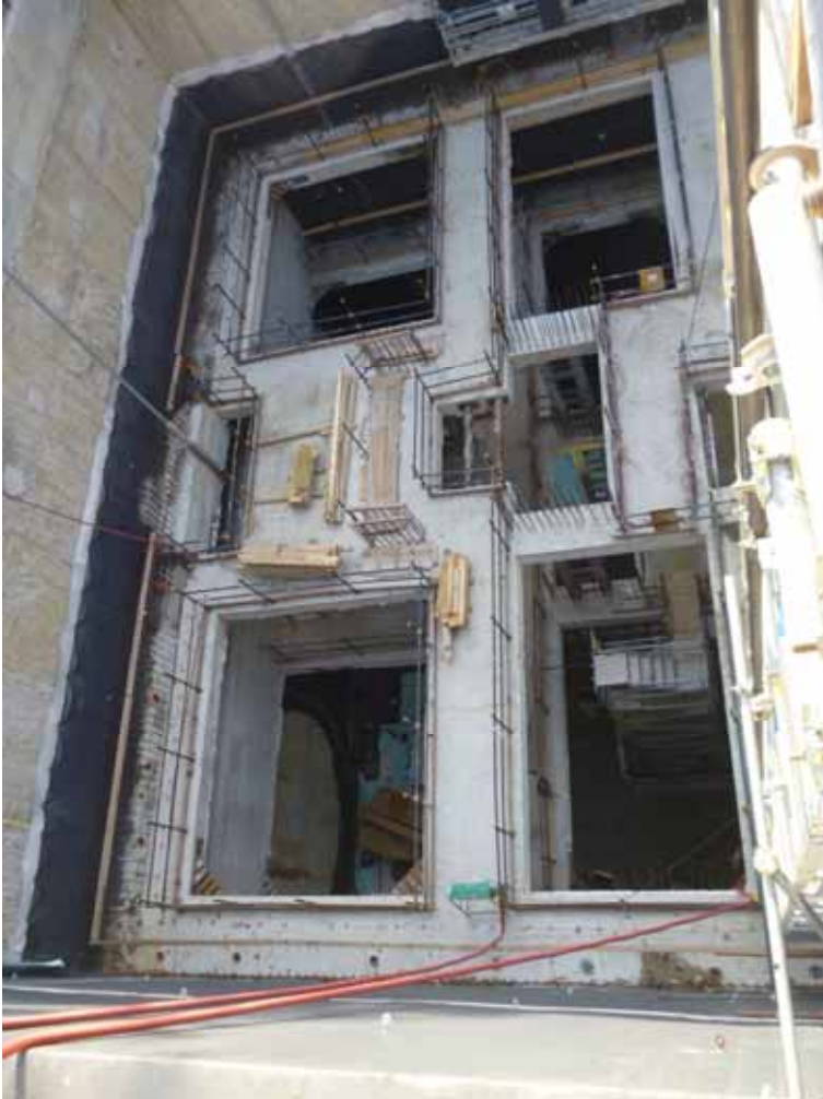
Fig. 9 Top-down decks: opening sizes
