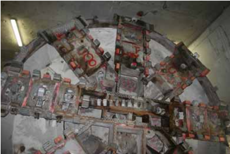
Fig. 7 Lotto station TBM Break-in
