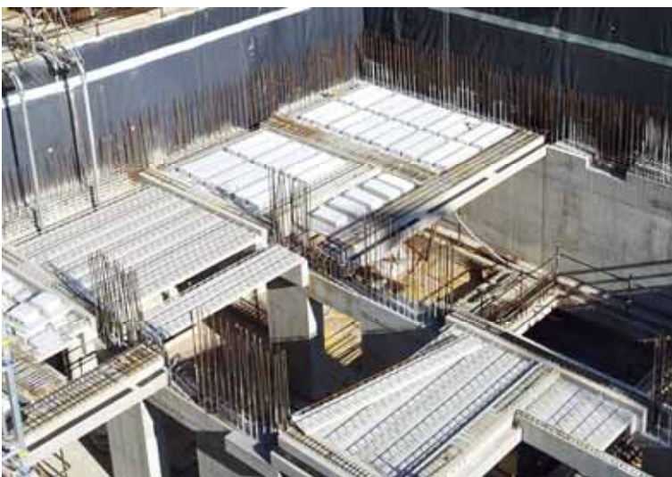
Fig. 12 Assembly phases of beams and slabs
