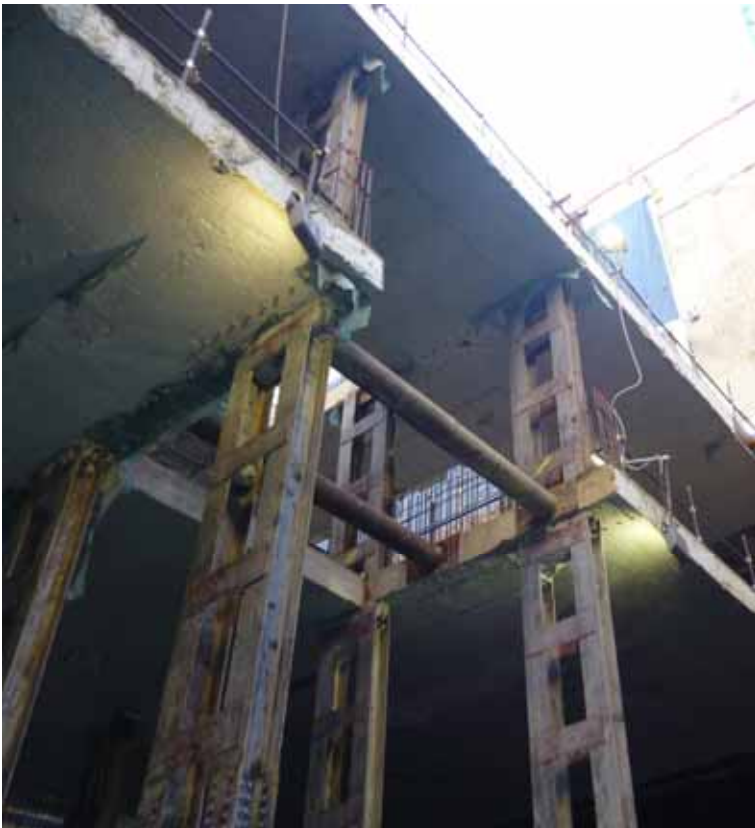
Fig. 10 Metal support columns, top-down decks
