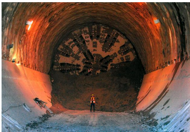
Figure 14. The EPB TBM "Martina" (15.62 m in diameter) has just completed the excavation of the first barrel of the "Sparvo" tunnel (A1 motorway between Bologna and Florence).
