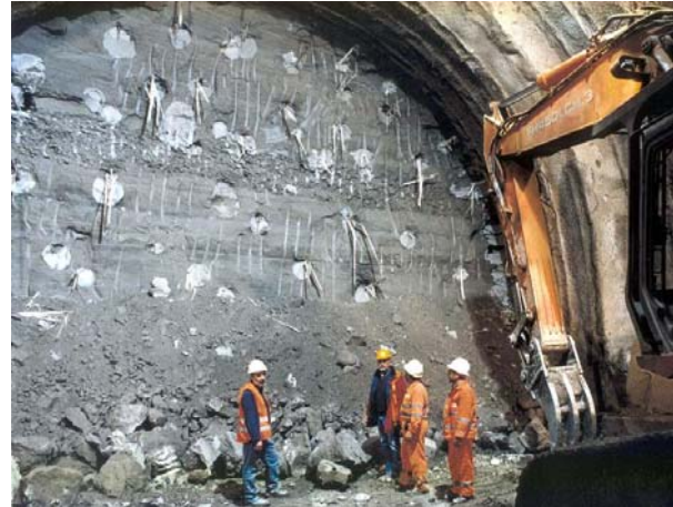
Figure 24. Firenzuola tunnel, the core-face improved with reinforced micro-jet (ground: clayey sands with pebbly intercalations, overburden: ~ 40 m).
