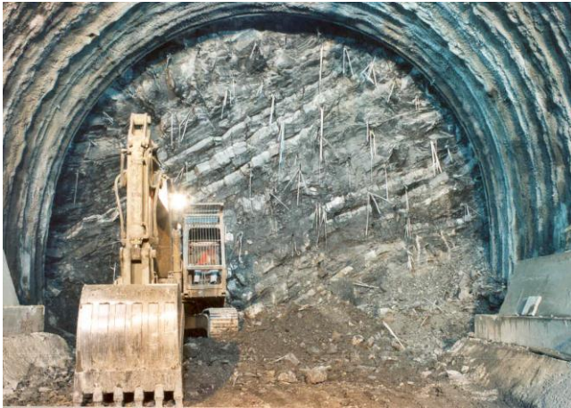
Figure 23. Monte Bibele tunnel, the core-face reinforced with fibre-glass elements (ground: Monghidoro flysh, overburden: ~ 200 m).
