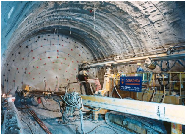
Figure 9. Core-face reinforcement execution – drilling
