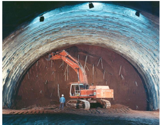
Figure 5. Core-face reinforcement in cemented sand
