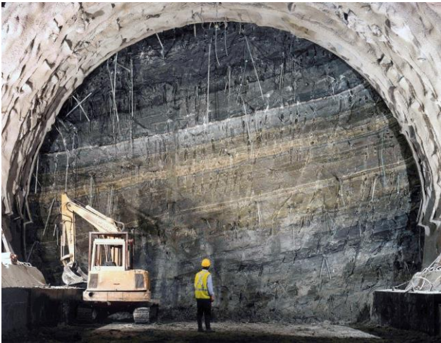
Figure 6. Core-face reinforcement in soft rock
