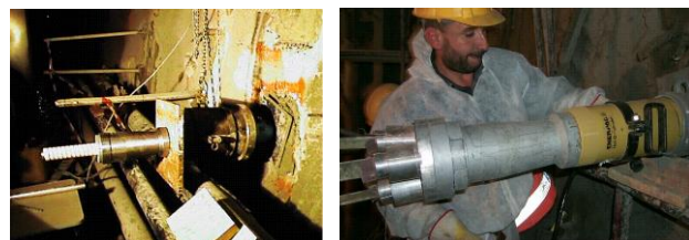
Figure 11. Fiber glass extraction test
