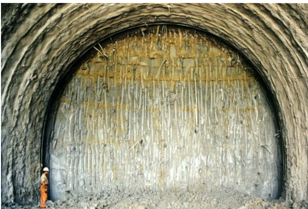
Figure 4. Core-face reinforcement in clayey materials
