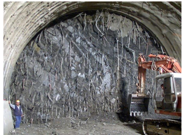
Figure 3. Core-face reinforcement in the ADECO-RS approach for tunneling
