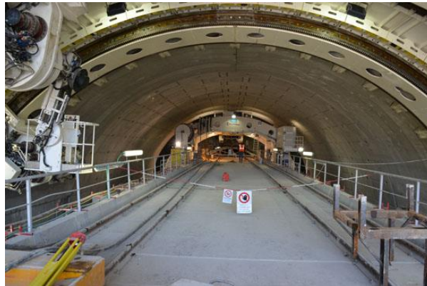
Figura 6. Montedomini tunnel: construction site area above the shield
