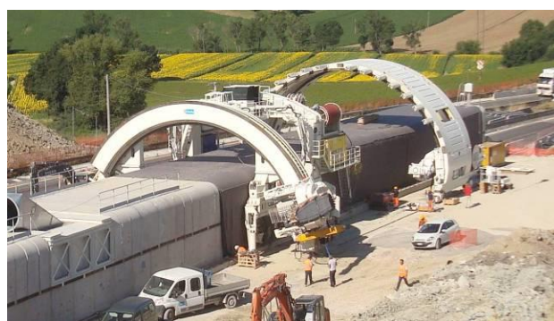
Figura 7. Montedomini Tunnel: the two machines used to widen the tunnel in the presence of traffic
