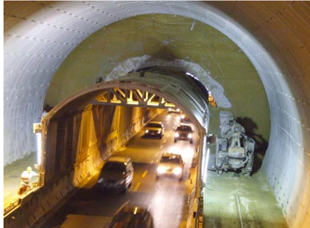
Figure 2. Nazzano Tunnel: traffic protected by the steel protection shield while the old tunnel is being widened
