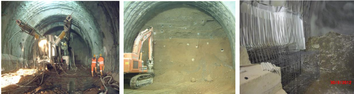
Figure 7. Main execution phases: grouting treatment, excavation and invert casting
