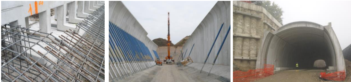
Figure 10. a) C&C Tunnel and temporary retaining structures
