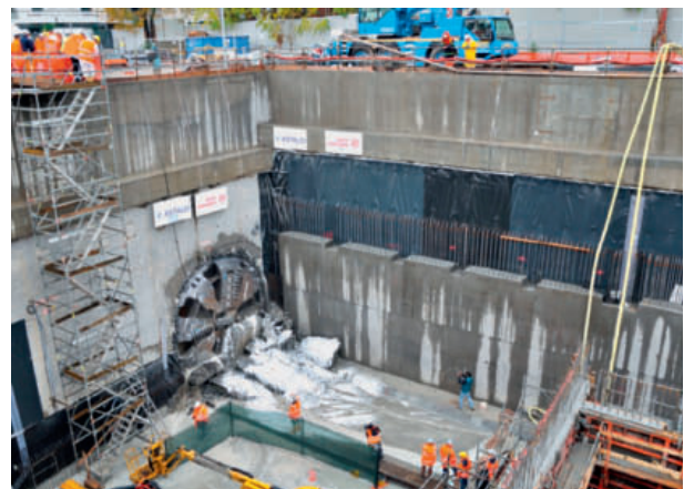
8 11.11.2014: arrivo TBM binario dispari a Forlanini FS 11.11.2014: arrival of TBM, odd track at Forlanini FS
