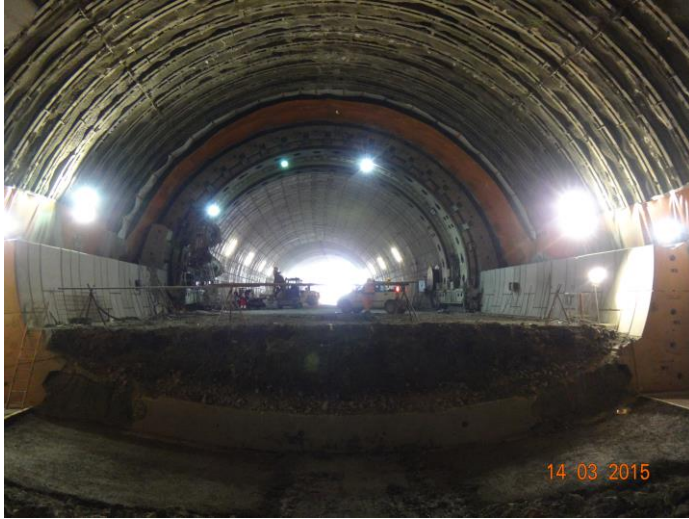
Figure 10. General view of the south bore of “Montedomini” tunnel during the widening works
