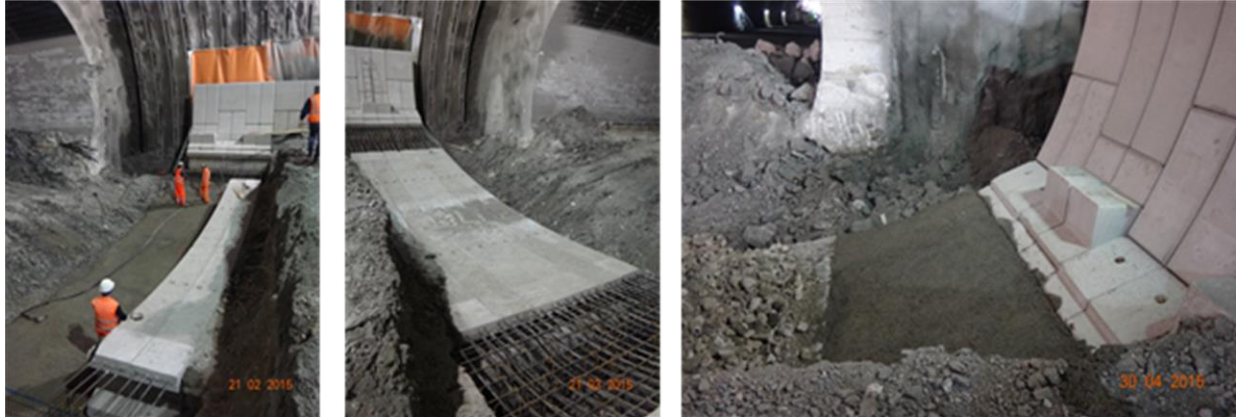
Figure 9. Placing of the prefabricated segment of the invert, reinforcing and placing of side completion casts
