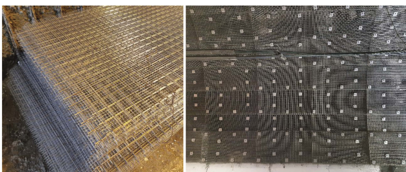
Figure 5. a) Double coupling layer nets; b) Anchoring net system by dowels.
