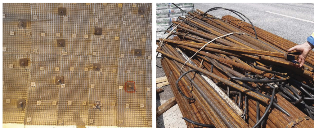
Figure 6. a) Reinforcement with bolts and nets; b) Detail of bolt anchoring.
