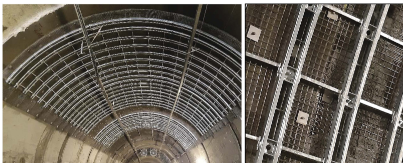
Figure 7. a) Reinforcement with steel ribs; b) Detail of coupled rectangular hollow steel profiles.
