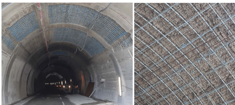
Figure 8. Intervention for reinforcement corrosion protection and concrete cover reconstruction.
