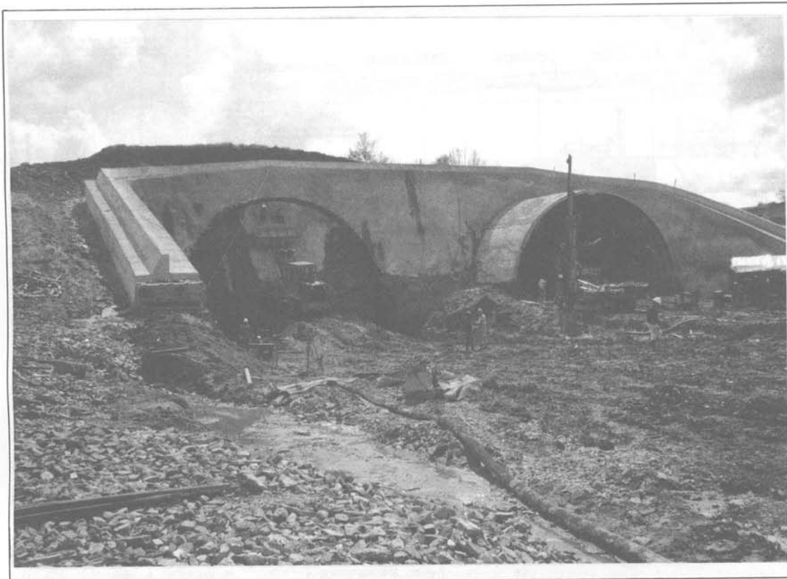
Fig. 3: Galleria "Rimazzano, imbocco Nord. Rimazzano tunnel North opening.
