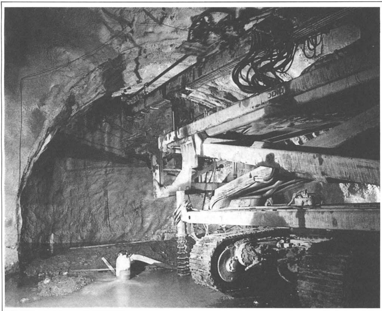
Fig. 3: Attrezzatura per il jet-grouting. Jet-grouting drilling machine.
