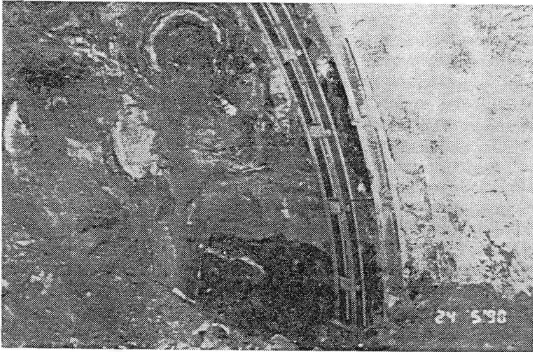
Photo 3 - San Vitale Tunnel: ground at the face (Argille Varicolori)
