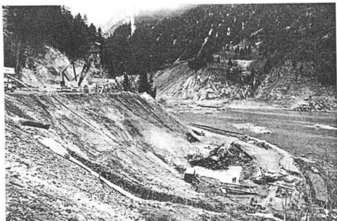
Figure 6 View of up-hill works for water inlets.
