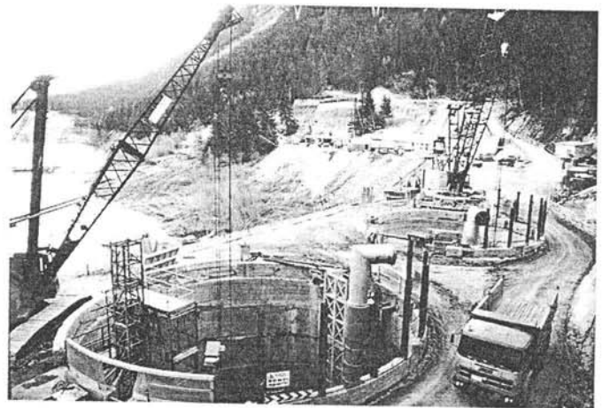
Figure 9 General view of the up-hill access shafts.
