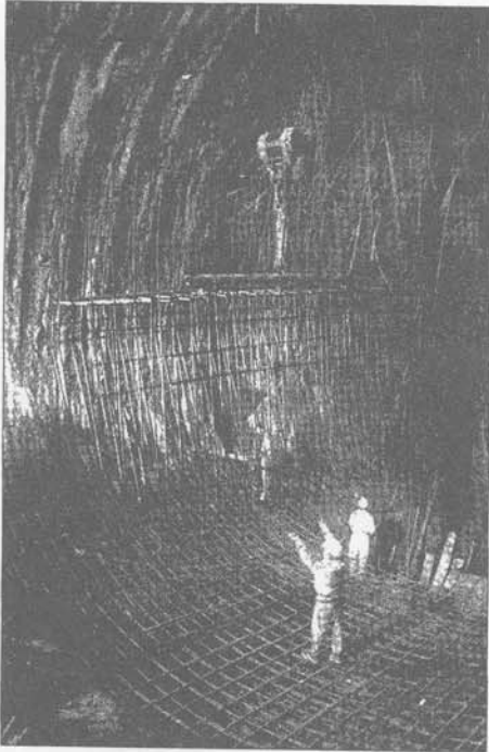
Tunnel Raticosa, renforcement des terrains
