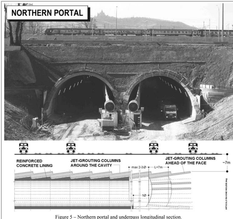
Figure 5 – Northern portal and underpass longitudinal section.
