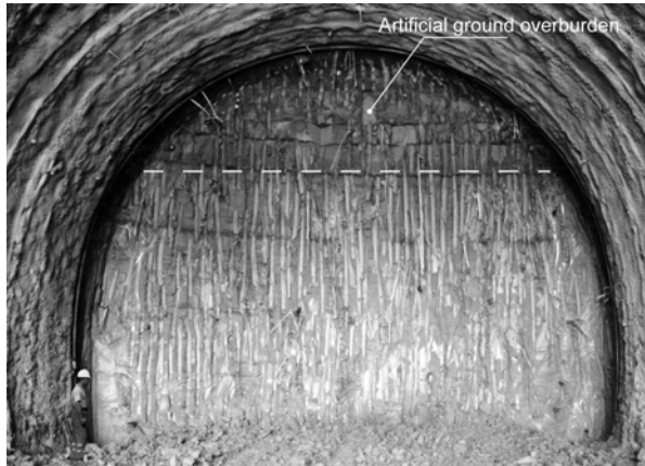
Figure 6. Borgo Rinzelli tunnel: the face during the advance under artificial ground overburden
