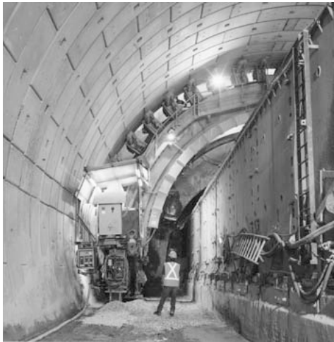
Figure 9. Erection of the prefabricated lining segments in pretressed r.c.
