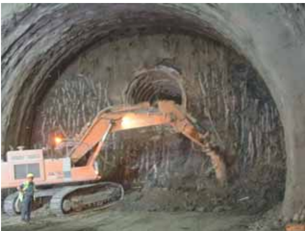
Photo 4 – Section type C2 – Full face tunnel advance
