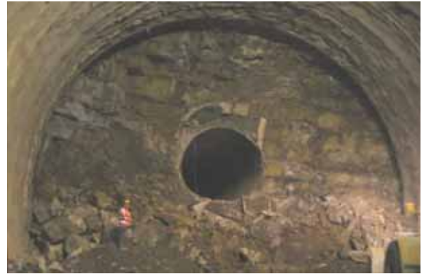
Photo 1 – North portal pilot tunnel
