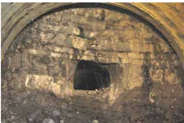
Photo 2 – Monte Cervarola Sandstones – Section type B0
