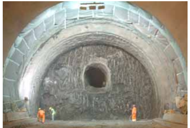
Photo 8 – Section type C2 – Final lining-face distance
