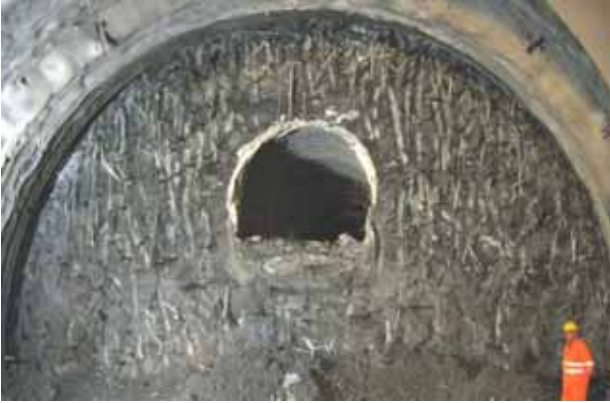
Photo 3 – Scaly Clays – Section type C2
