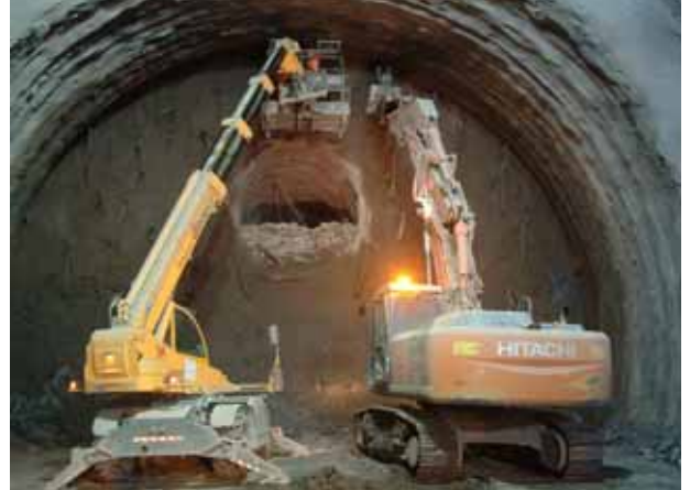
Photo 5 – Section type C2 – Placing steel ribs
