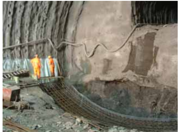
Photo 6 – Section type C2 – Reinforcing and casting the tunnel invert
