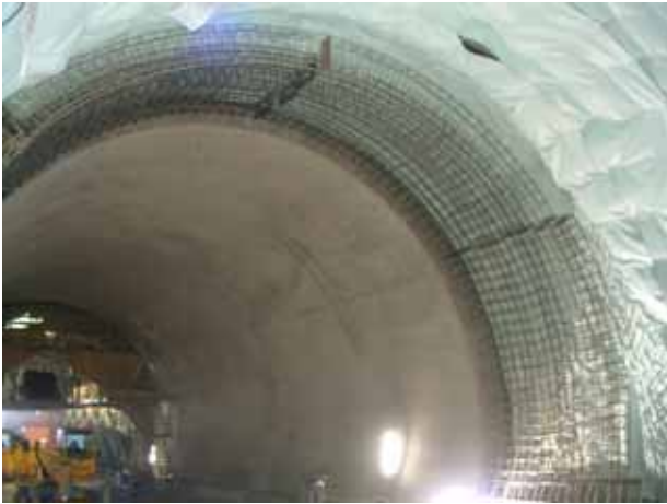
Photo 7 – Section type C2 – Casting the final lining
