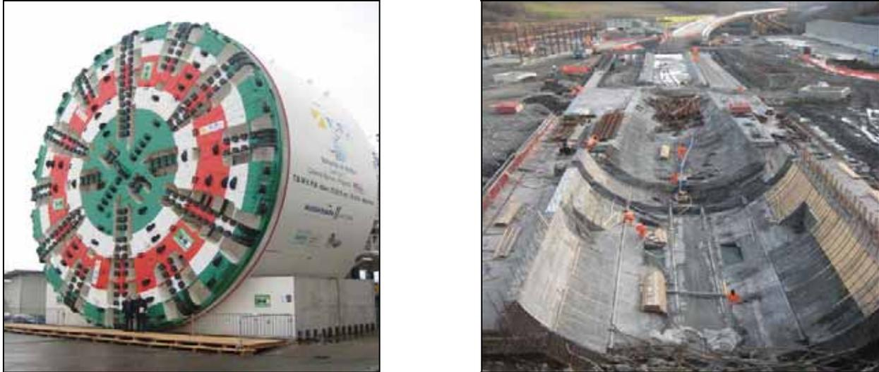
**Fig. 6** - Sparvo EPB-TBM (named "Martina") and the portal on the Florence side
