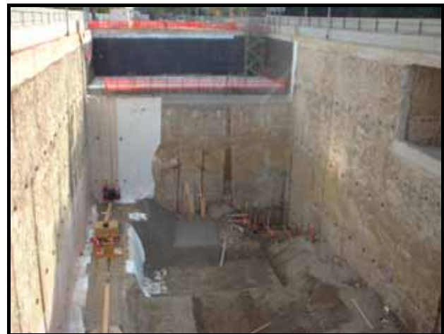
Figure 10 - Ponale station pit
