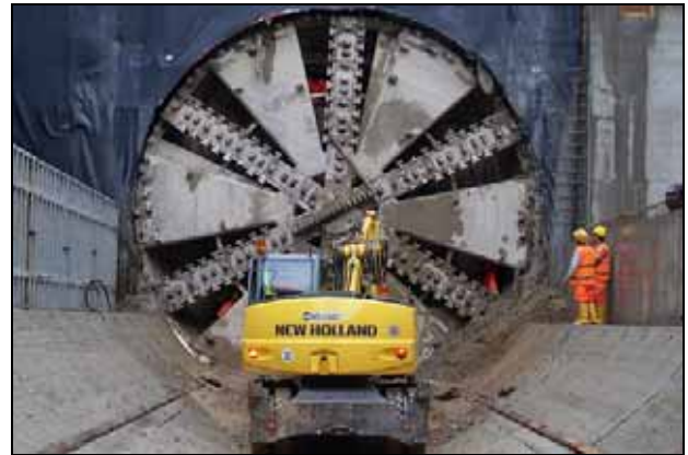
Figure 5 - TBM before passing through the excavated station
