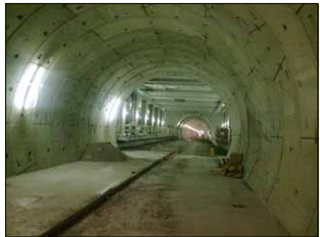
Figure 6 - Artificial TBM bored tunnel
