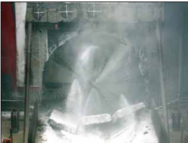
Figure 4 - Arrival of the TBM at Istria station (20.04.2009)
