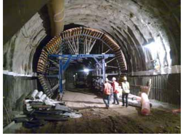
Figure 9 - Conventional excavation (widening at Zara Station)
