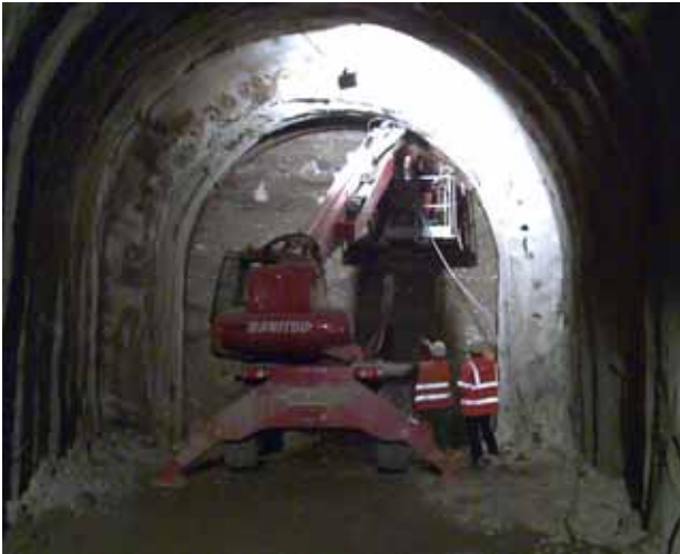
Figure 7 - Conventional excavation (single track tunnel)
