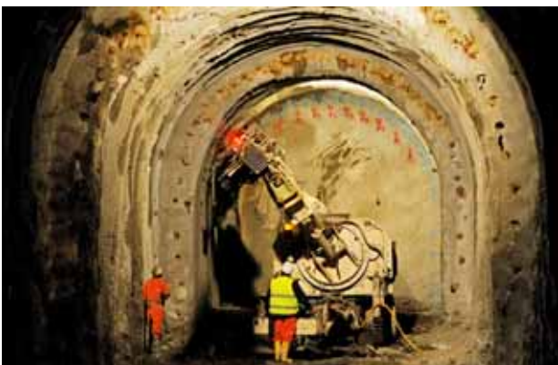
Figure 8 - Conventional excavation (single track tunnel)
