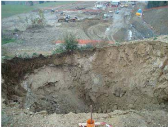
Figure 6 Fuciello Tunnel: collapse at the north portals of 11-11-2008
