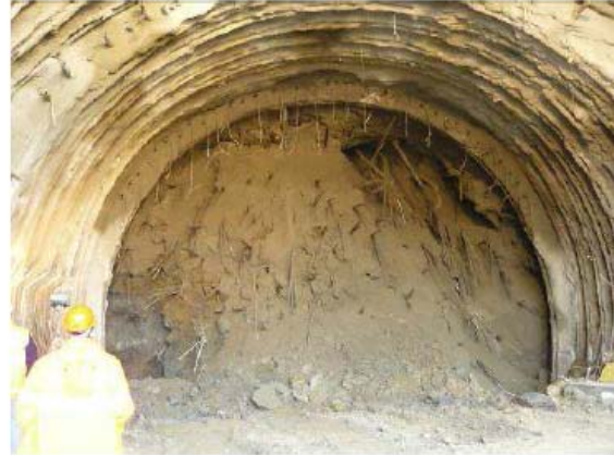
Figure 6 Fuciello Tunnel: collapse at the north portals of 11-11-2008
