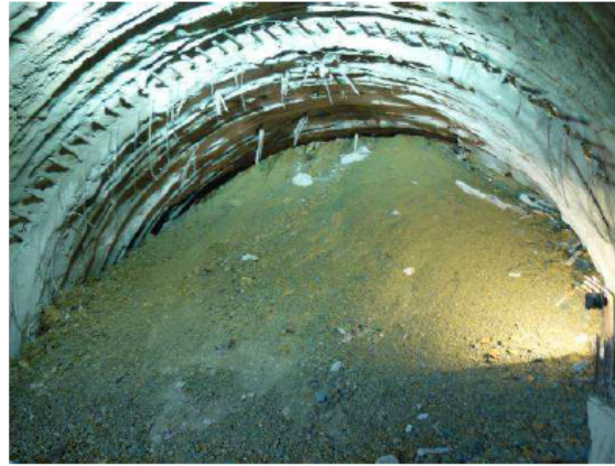
Figure 5 – Cerzone Tunnel: collapse at north portals of 26-09-2008
