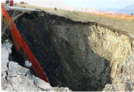
Figure 5 – Cerzone Tunnel: collapse at north portals of 26-09-2008
