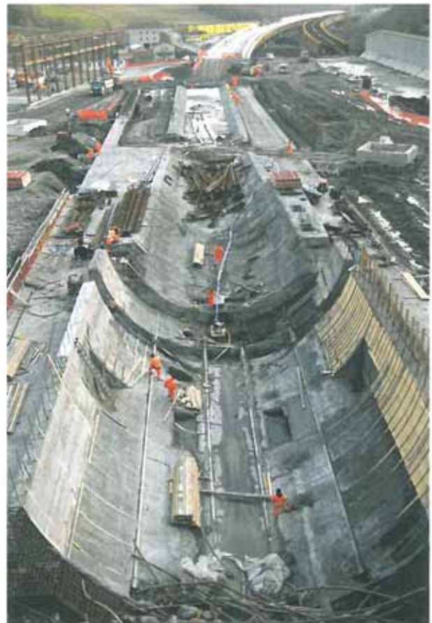
8b Facilities for housing the EPB TBM at the portal on the Florence side
