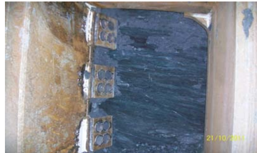
Figure 3. Km. 1+525 Face Condition
