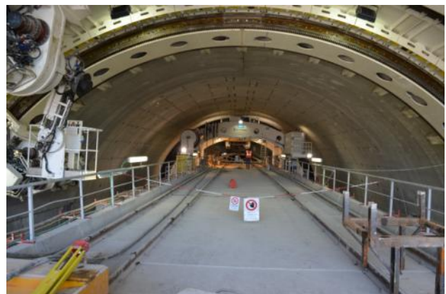
Figure 9. Montedomini tunnel: construction site area above the shield
