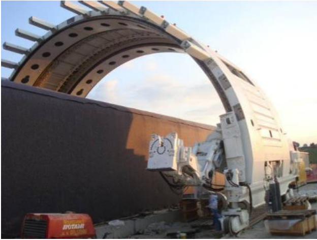
Figure 12. Segment erection machine
