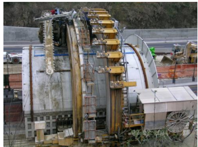
Figure 4. Nazzano tunnel: the Multifunction Machine
