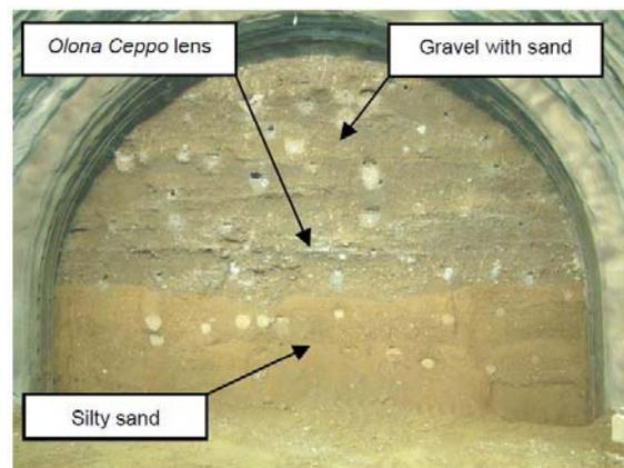
Figure 6. Geological face mapping.
