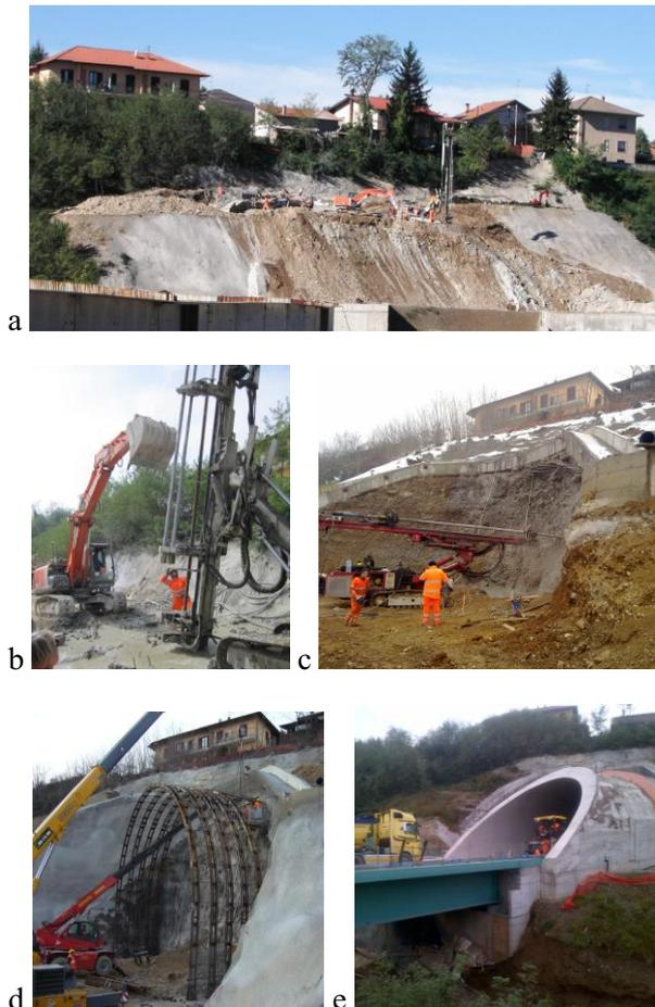
Figure 16. The executive phases: a) working area, b) treatment execution, c) core face treatment, d) jig construction, e) cast-in place portal.
