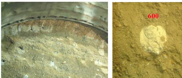
Figure 8. “Mono-fluid Jet-grouting” (600 mm).
