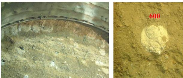
Figure 8. “Mono-fluid Jet-grouting” (600 mm).
