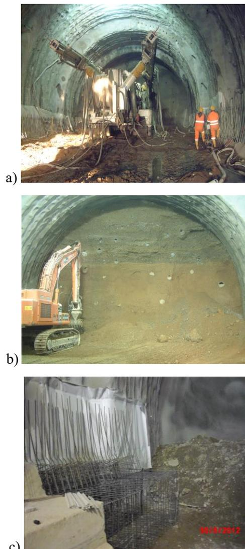
Figure 11. Main execution phases: a) grouting treatment, b) excavation, c) invert casting.
