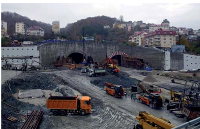
Fig. 8 – North portal during construction.
