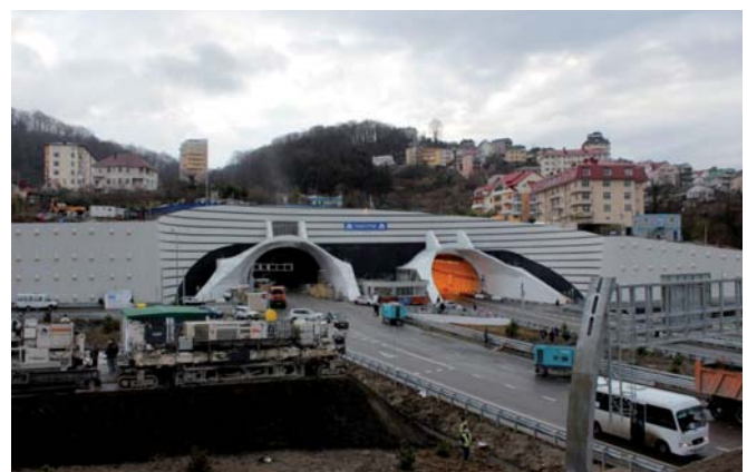
Fig. 9 – North portal almost finished.
