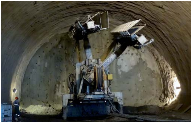
Fig. 10 – Core-face reinforcement by using a tunnelling rig machine.
