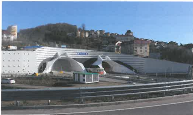
Fig. 4. View of the Sochi North Portal showing densely inhabited areas
