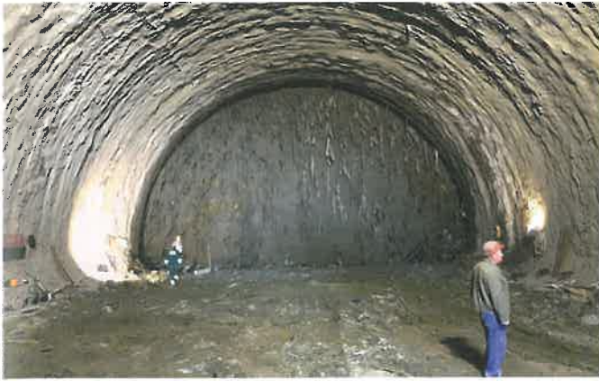
Fig. 7. View of the tunnel face showing the core-face stabilization measures
