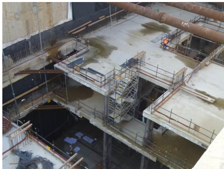
Figure 4. Construction stages: top-down slabs
