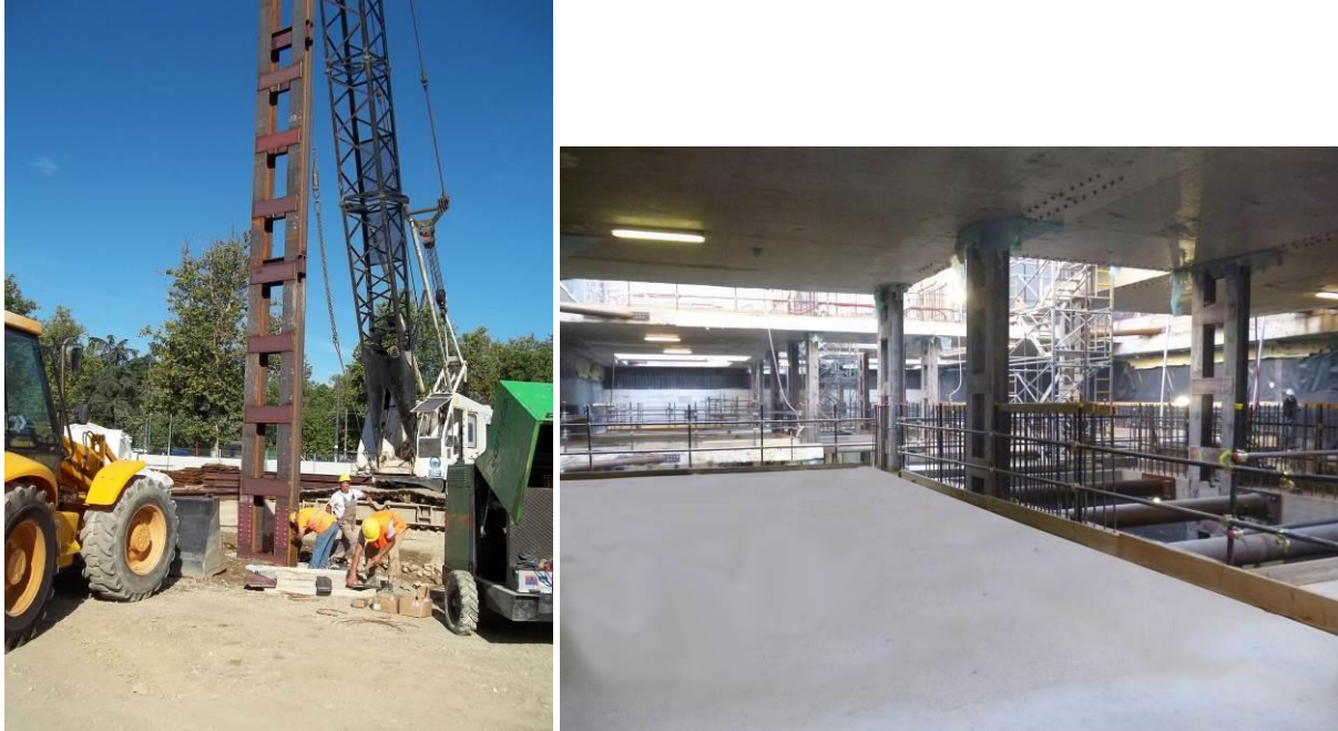
Figure 5. Temporary steel pillars
