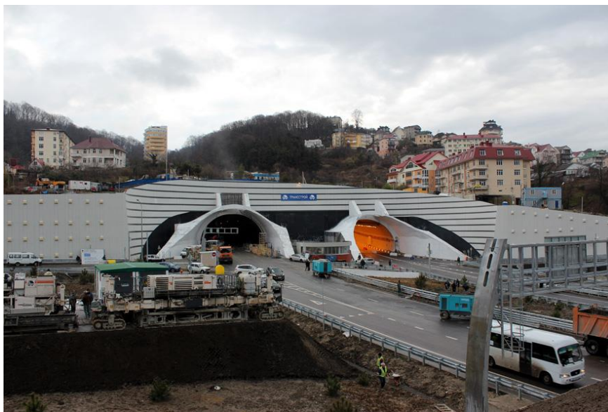
Figure 6. North portal almost finished
