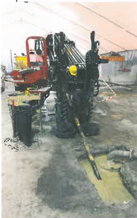
Left: A horizontal directional drilling rig
