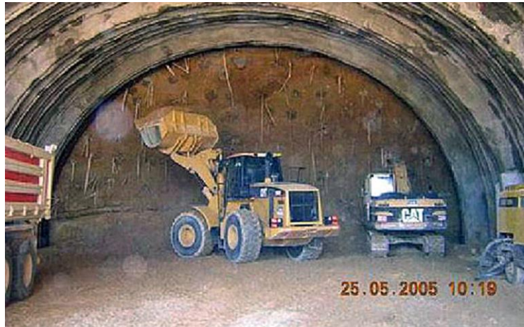
Figure 24: Phase of demolition of the face
