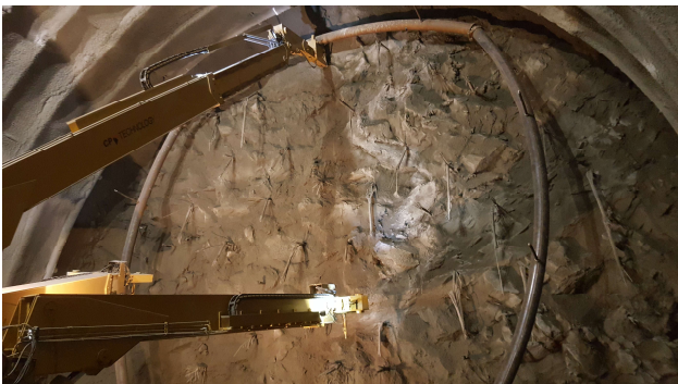
Figure 6. Tubular Arch opening.
