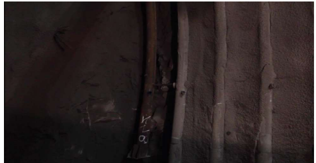
Figure 7. Tubular Arch connection by insertion of the bracing elements.
