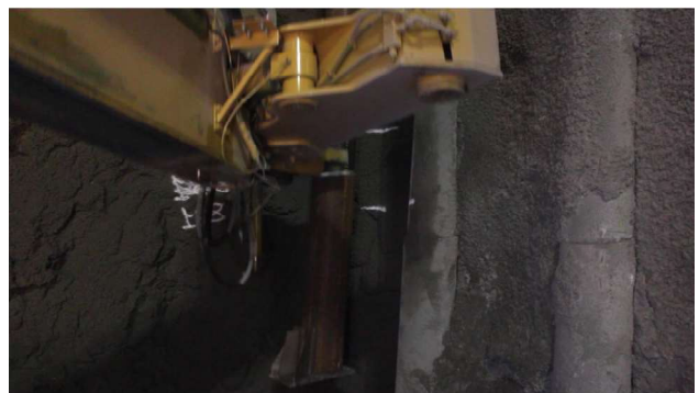
Figure 8. Tubular Arch foot extension and positioning.
