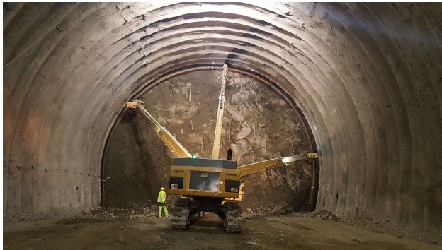
Figure 9. Tubular Arch installation by EKIP 2104.
