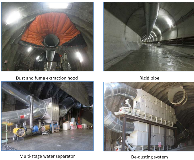
Figure 10 - Components of Extraction ventilation system
