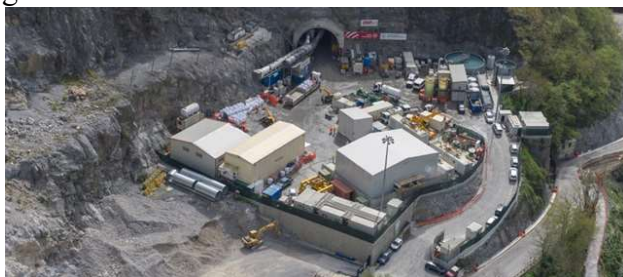
Figure 13. Cravasco Site: aerial view
