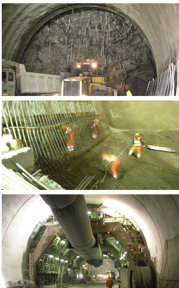
Figure 7. ADECO Construction process – Main phases.
