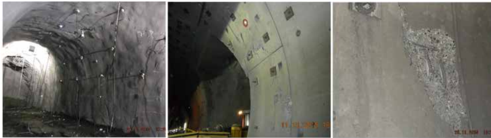
Figure 18. Cracks on the preliminary lining of the shelters and segmental linings
