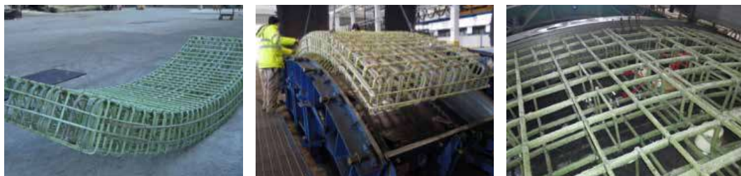
Figure 1. GFRP reinforcement for segment linings
