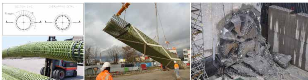
Figure 4. GFRP “soft eye”
