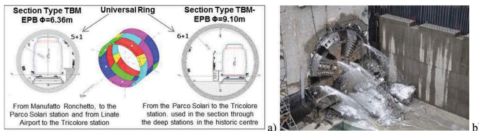
Figure 2. a) TBM Sections type; b) Forlanini Railway Station: TBM breakthrough odd track.
