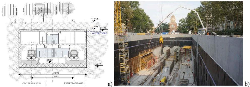
Figure 3. Argonne Station: a) Detail of the reinforced concrete piling; b) general view.
