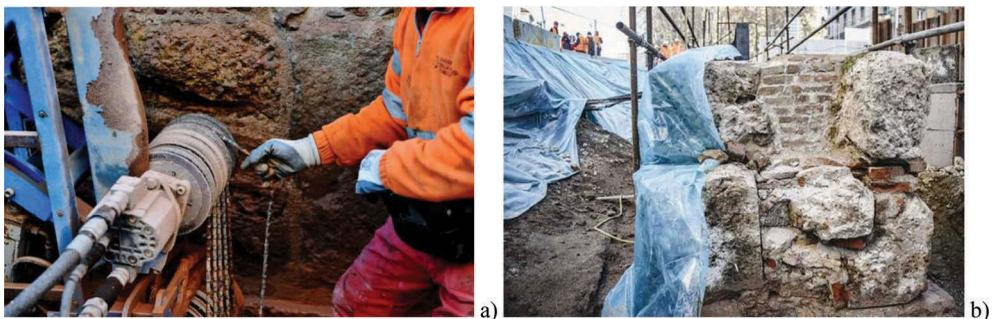
Figure 10. a) Diamond wire used for wall cutting; b) Roman wall detail.
