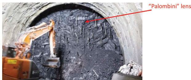
Figure 10. “Argille a Palombini” Formation – claystone schist with limestone lens.
