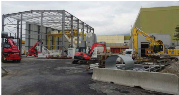
Figure 9. Point 5 site works at September 2018 – Surface works.
