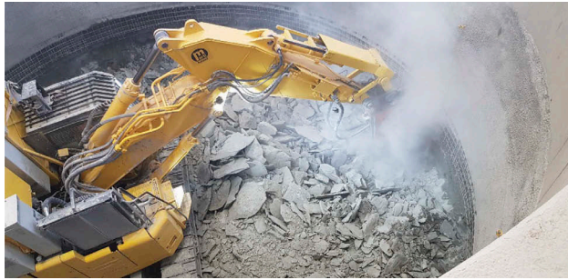
Figure 8. Point 1 Shaft excavation.
