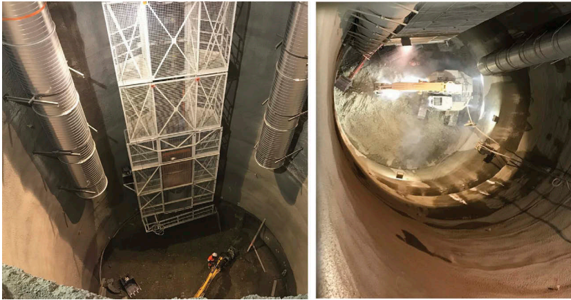
Figure 11. Point 5 – Shaft excavation (2).
