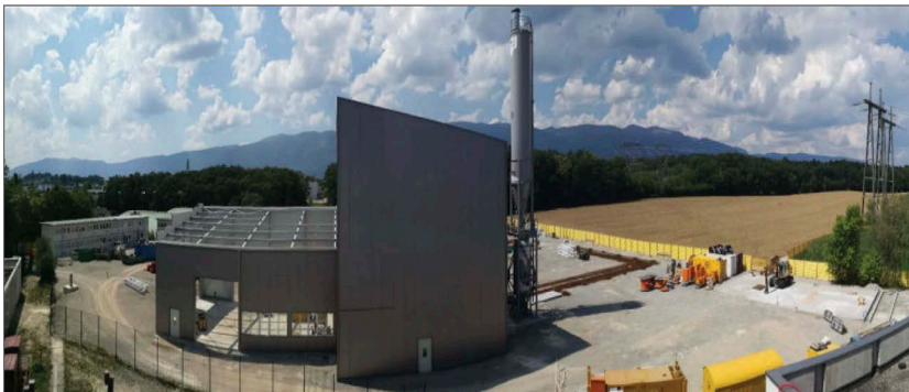
Figure 7. Point 1 site works in August 2018 – Surface works.
