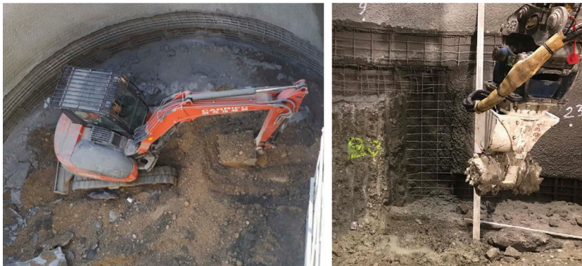
Figure 10. Point 5 – Shaft excavation (1).
