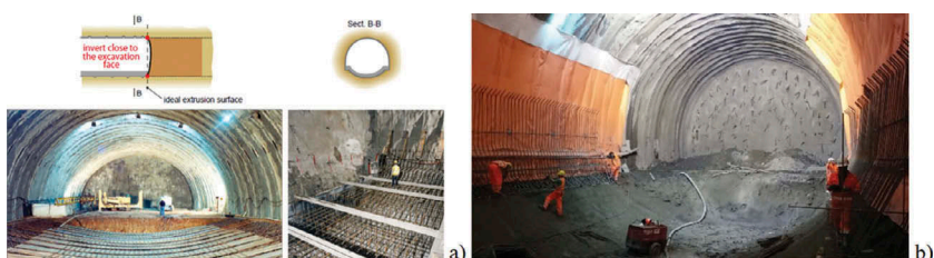
Figure 6. Example of conservation technique: a) Invert; b) advance core GFRP reinforcement and invert.
