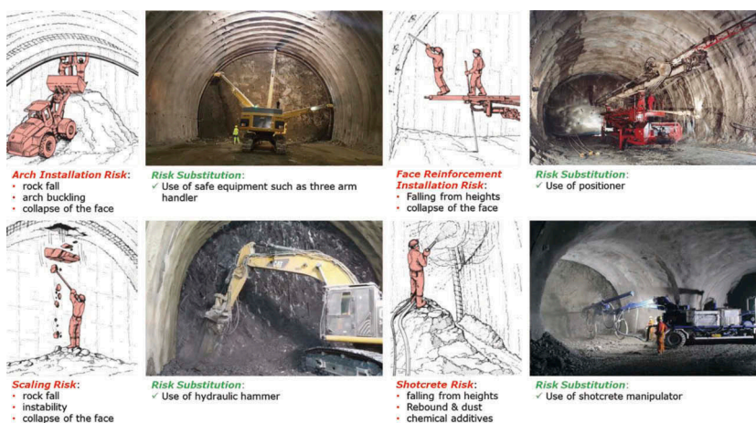
Figure 11. Example of risk reduction through the application of a full-face excavation method.
