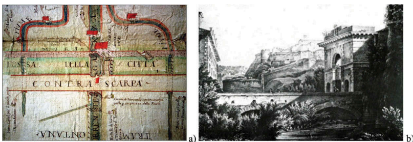
Figure 3. Porta Pile: a) Iseppo Cuman Map (1667, Brescia, Archivio di Stato, ASC 999); b) Stone bridge, built in 1818, found during metro line construction work (engraving of Fausto Pernici (1840–1850)).
