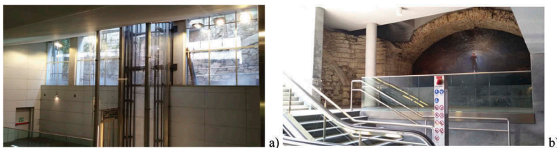
Figure 7. a) Large section of Venetian wall (sixteenth-century) visible along the south side of the station; b) nineteenth-century stone's bridge, upper atrium view.
