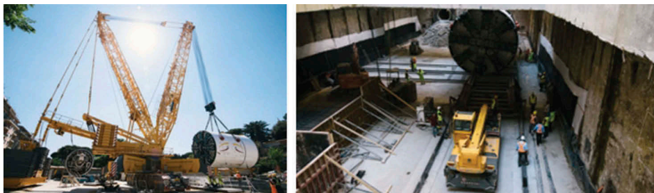
Figure 5. TBM job site in shaft 3.3.
