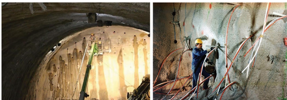
Figure 4.29 Fibreglass element installation (Lunardi, 2008).
