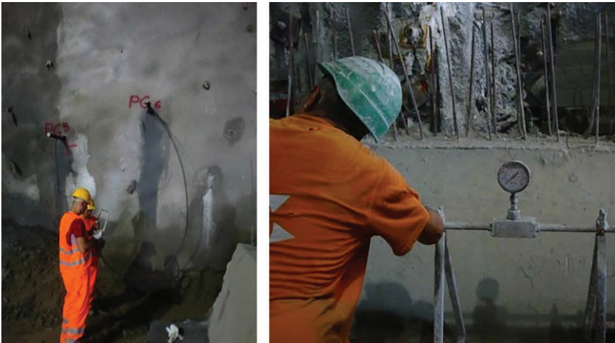
Figure 4.30 Fibreglass element grouting.
