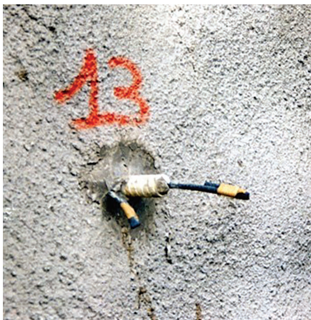
Figure 4.31 Detail of fibreglass reinforcement grouted with cement mixture.
