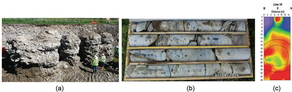
Figure 4.50 (a) Direct site inspection; (b) coring of treated soil; (c) cross-hole tests.
