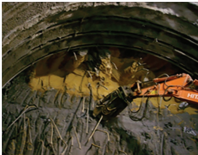
Figure 4.17 Detail of scraper-excavating machines, the drilling pipes are first bent by the excavator and then cut off with a robust shears that is driven by the excavator pivoting arm.
