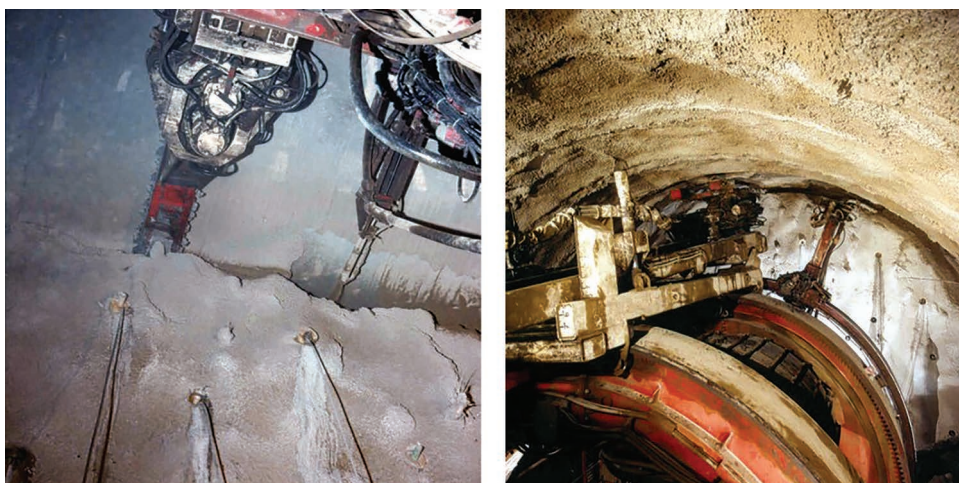
Figure 4.65 Cavity preconfinement by means of full-face mechanical precutting: execution and filling of the pre-cut (Lunardi, 2008).
