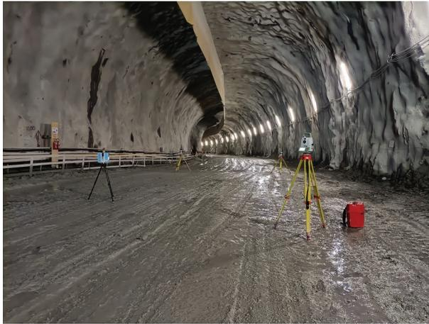
Figure 5.3 Application example of the laser scanner in tunnel construction. (Courtesy of Leica Geosystems AG.)
