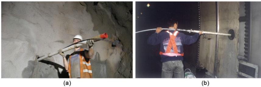
Figure 5.15 Example of incremental extensometer measurements in tunneling. (Courtesy of GD Test S.r.l.)
